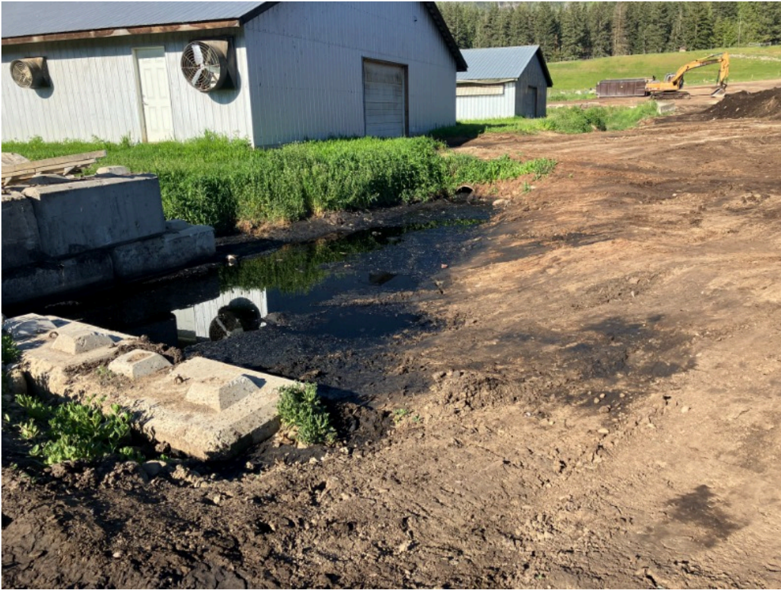
Photo 3. Unlined ditch to collect and direct runoff and excess precipitation from the compost storage area to the lined water containment.
