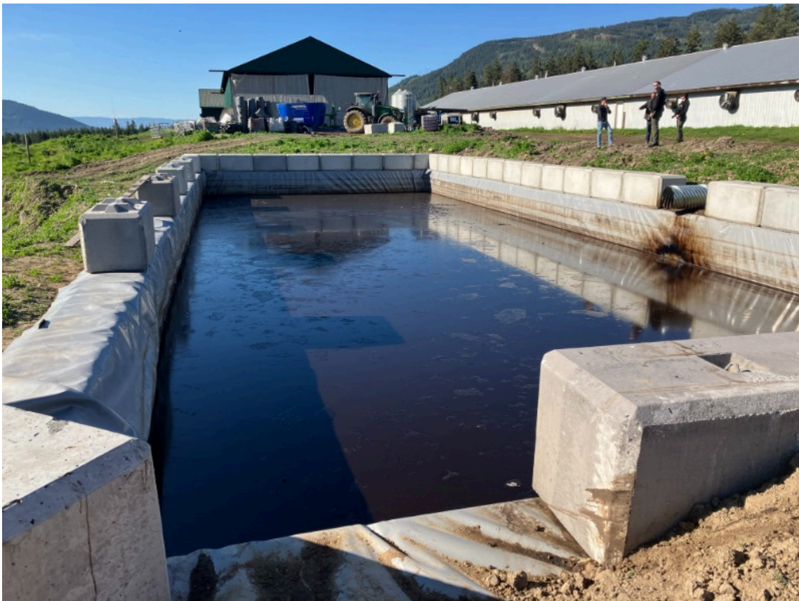
Photo 4. Lined water containment to collect runoff and excess precipitation from the compost storage area.
