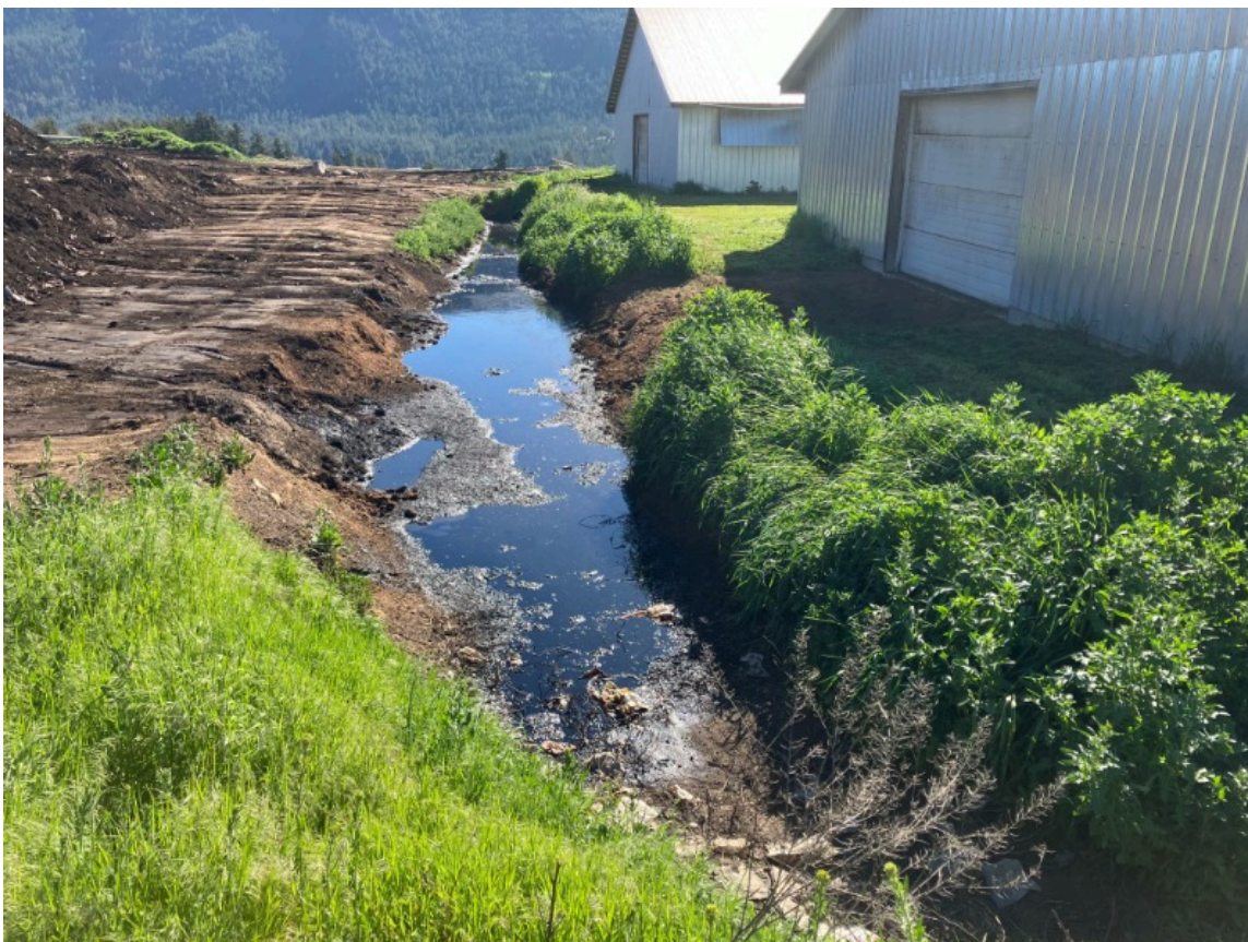
Photo 2. Unlined ditch to collect and direct runoff and excess precipitation from the compost storage area to the lined water containment.
